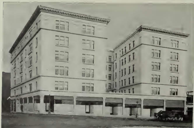
FRANKLIN BUILDING, SEATTLE, WASH. Walls of white enamel brick with terra cotta trim. Brick furnished by the American Enamelled Brick & Tile Co.
